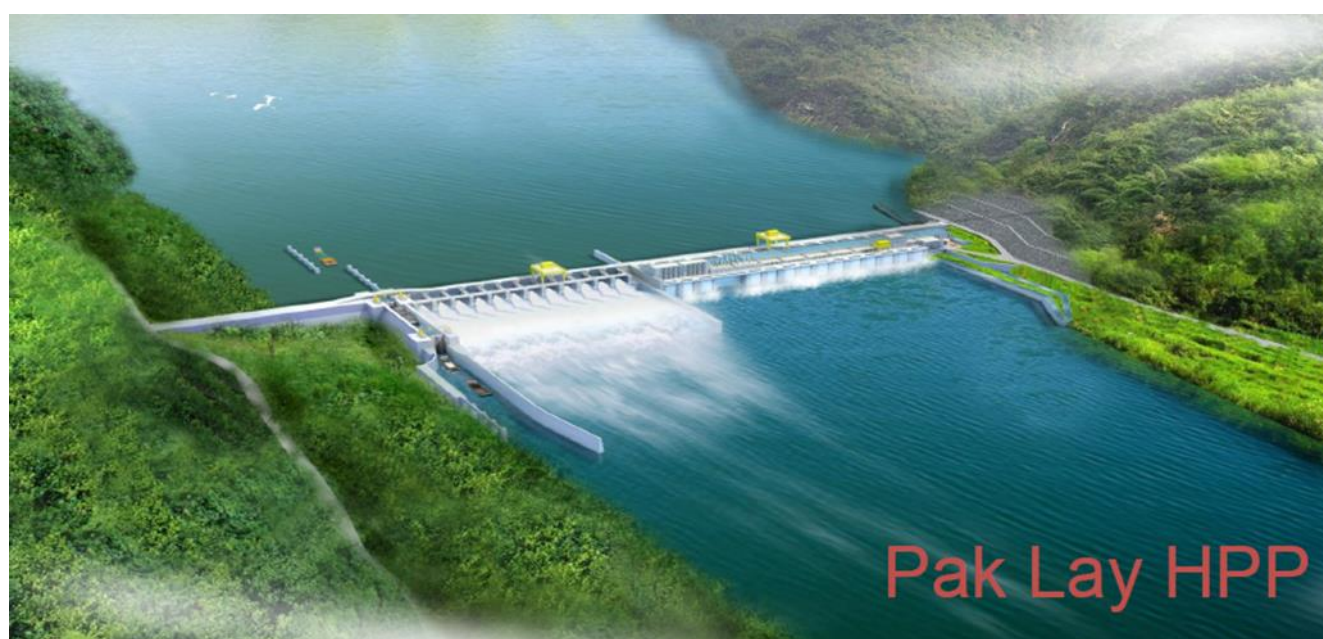
Figure 5: Pak Lay HPP General Overview.
