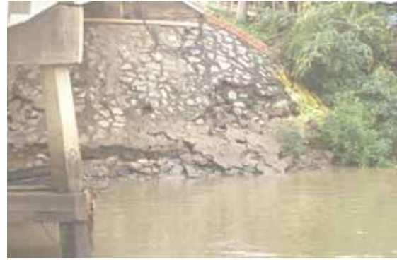
Figure 2.4 Examples of damage due to floods; damage to an unpaved road (left) and damage to a bridge abutment (right).
