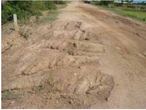
Figure 2.4 Examples of damage due to floods; damage to an unpaved road (left) and damage to a bridge abutment (right).
