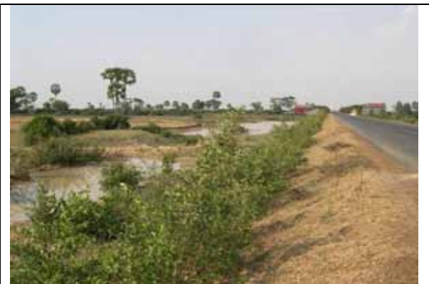
Figure 5.5 NR11 at the spillway.
