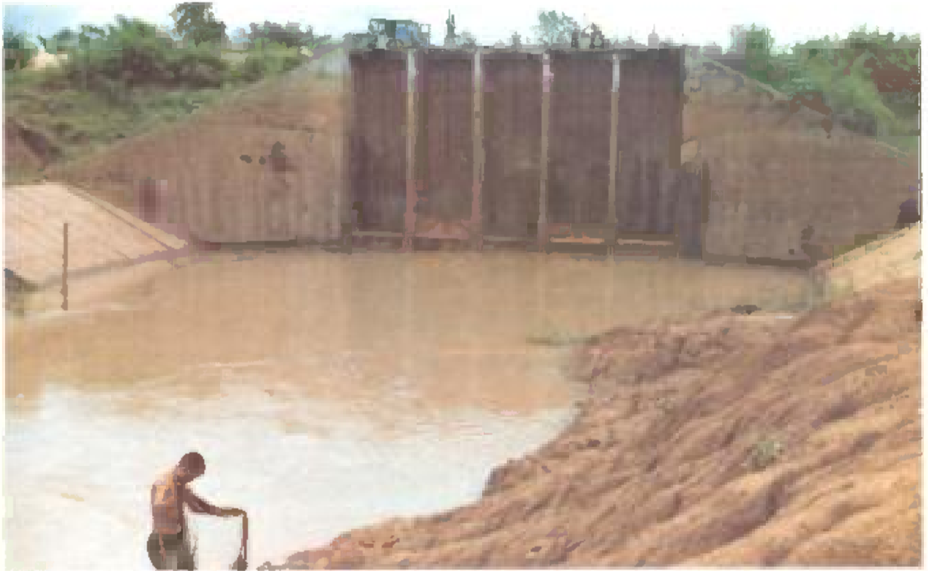
Part of the flood protection and reclamation of swamp and marshland in the Vientiane Plain involves the rehabilitation of flood control structures. Above, the Houei Mak Hiao regulator is shown after rehabilitation of the damaged trash racks and gates. Below, the Houei Van Vard flood control structure is shown following the installation of new flap gates
