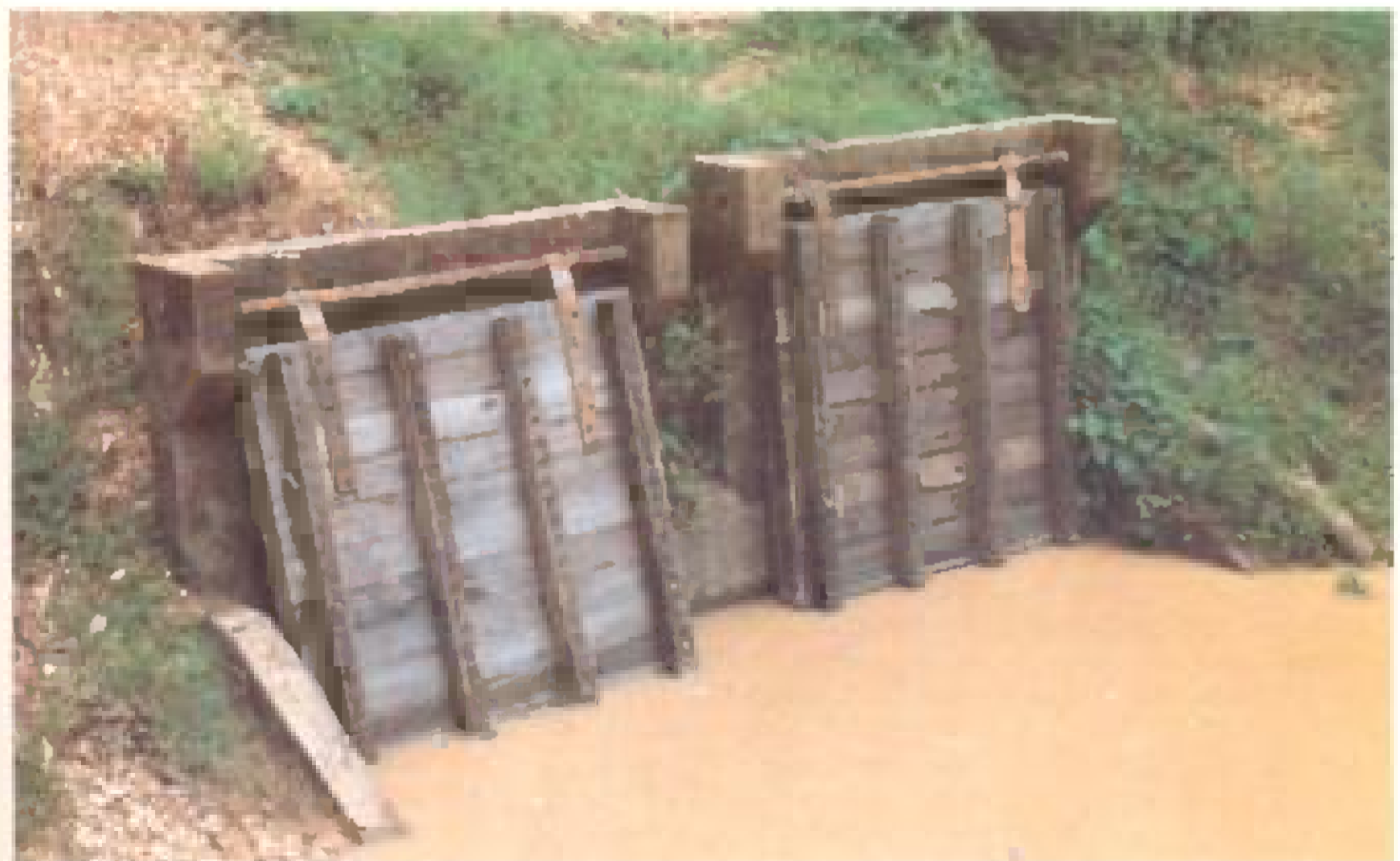
Part of the flood protection and reclamation of swamp and marshland in the Vientiane Plain involves the rehabilitation of flood control structures. Above, the Houei Mak Hiao regulator is shown after rehabilitation of the damaged trash racks and gates. Below, the Houei Van Vard flood control structure is shown following the installation of new flap gates
