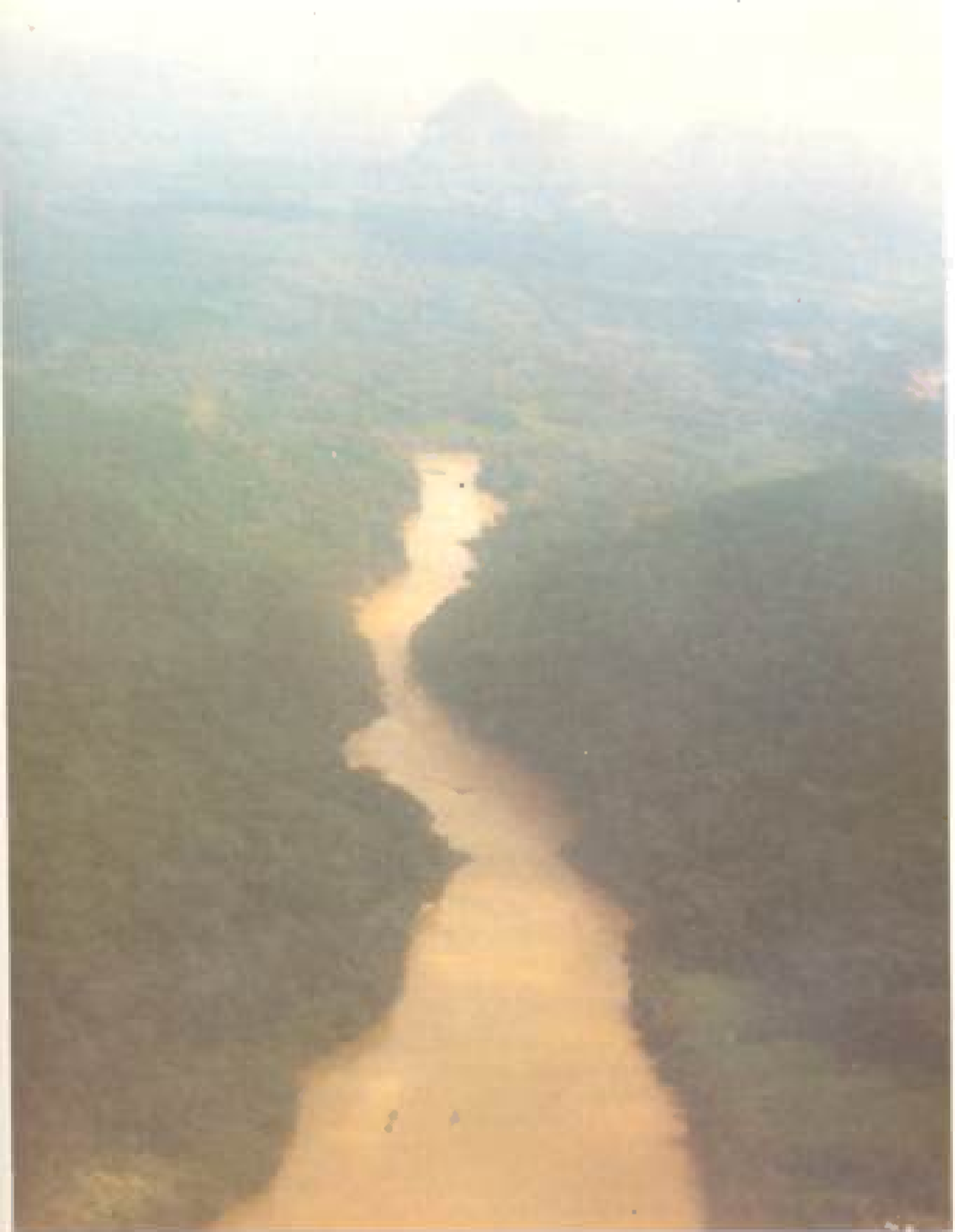
An aerial view of the proposed No 1-2 dam site on the Nam Theun River in the Lao PDR
