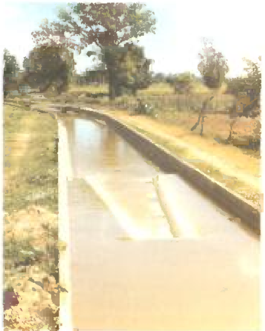
A duckbill weir in operation at the site of the water management support programme project in northeast Thailand. This type of weir allows more effective control of the flow and volume of water in an irrigation canal.
