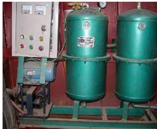
Figure 22: Oil-water separator
