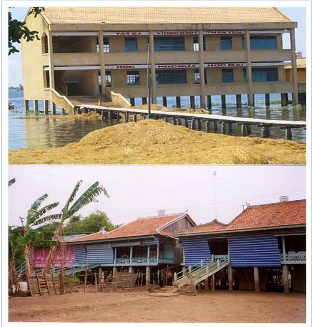
Figure 2-5 Flood ‘proofing’ in the Viet Nam Delta – school (top) and domestic property (bottom) raised on concrete columns.
