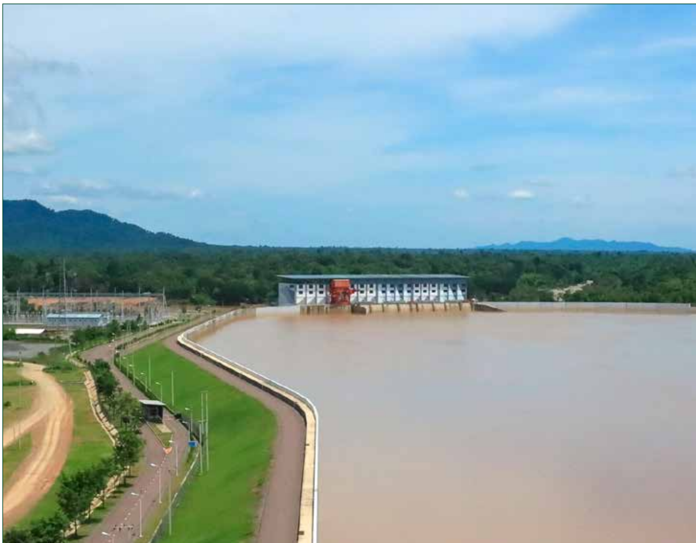
Don Sahong Dam, part of the second hydropower project on the mainstream of the Lower Mekong. The project is located in the Siphandone area of Champasak province – less than two kilometres upstream from the Cambodia-Lao border.
